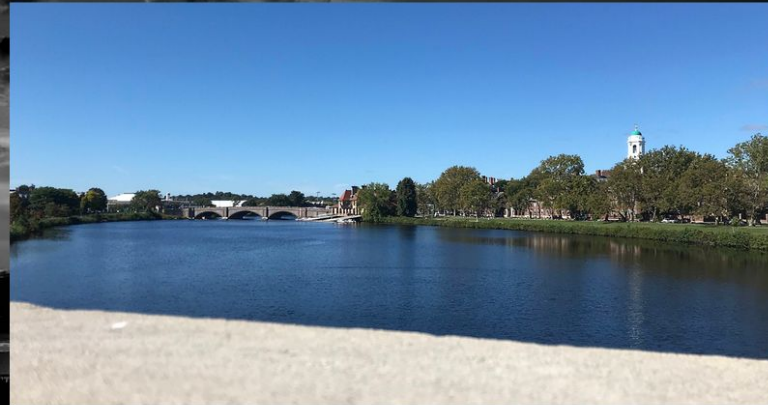
Weeks Bridge during the day.
